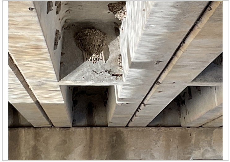
Delam to diaphragm @ unit 6.
