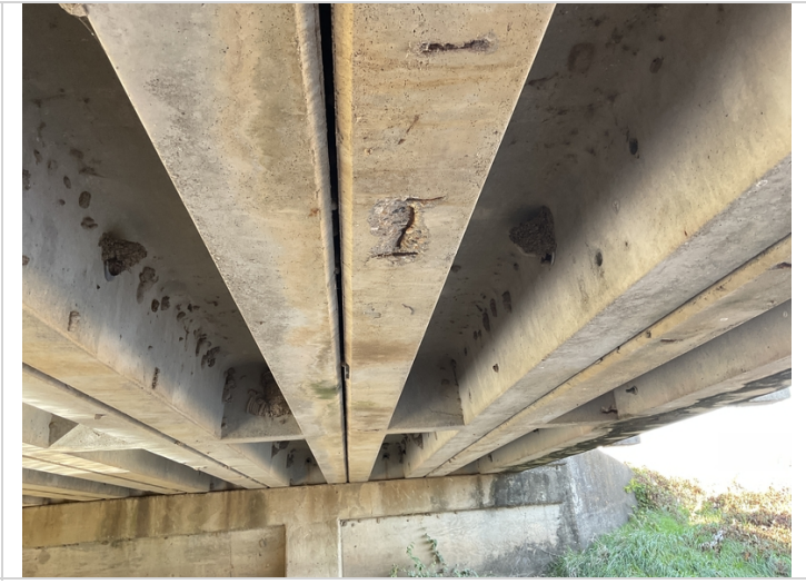
Spall with rebar exposed to unit 1, 2 , & 8.
